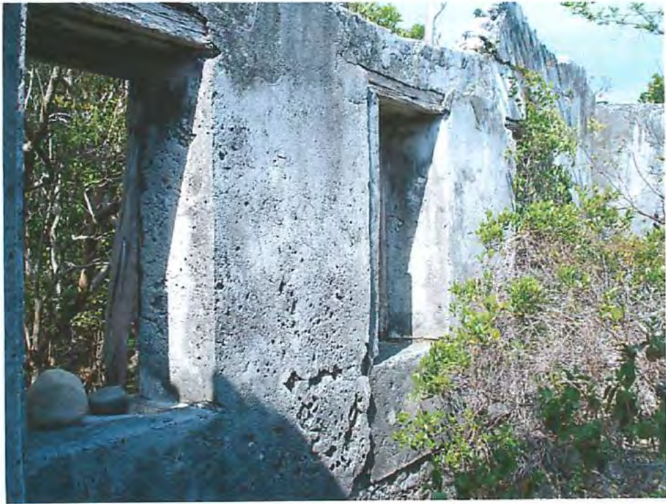
Figure 60, Barque Bay Structure 5, interior of north wall toward northeast
