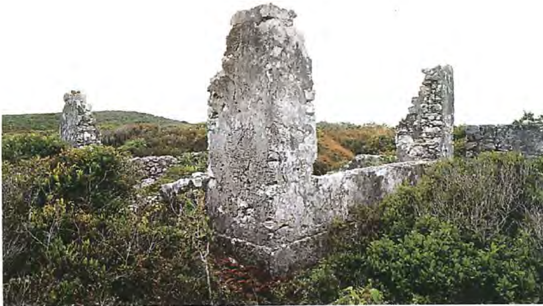
Figure 19, Lantern Head Structure 1 toward southwest from front yard. Southeast corner of Structure 2 is visible at far right.
