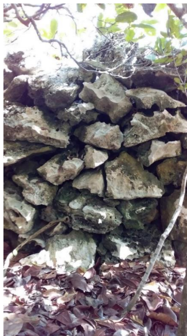
Figure 7.172. View of ruins at Barque Bay site
