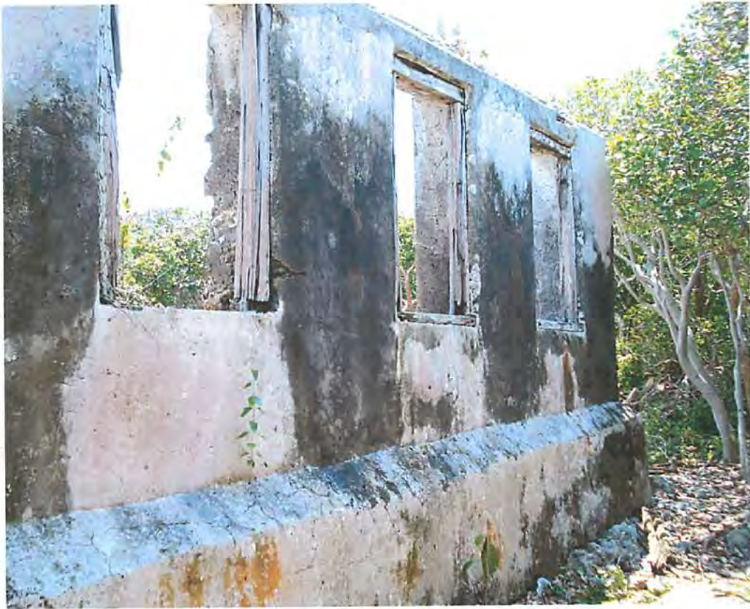
Figure 56, Barque Bay Structure 4, detail of north facade, toward southwest
