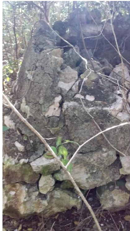
Figure 7.171. View of ruins at Barque Bay site
