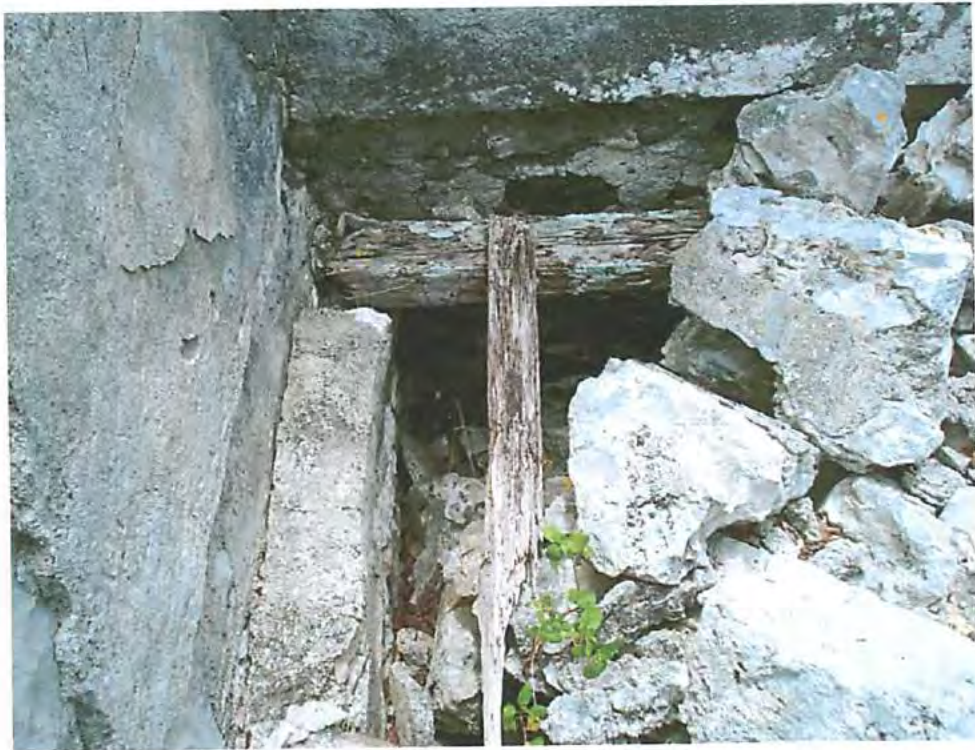
Figure 61, Barque Bay Structure 5, detail of floor joists
