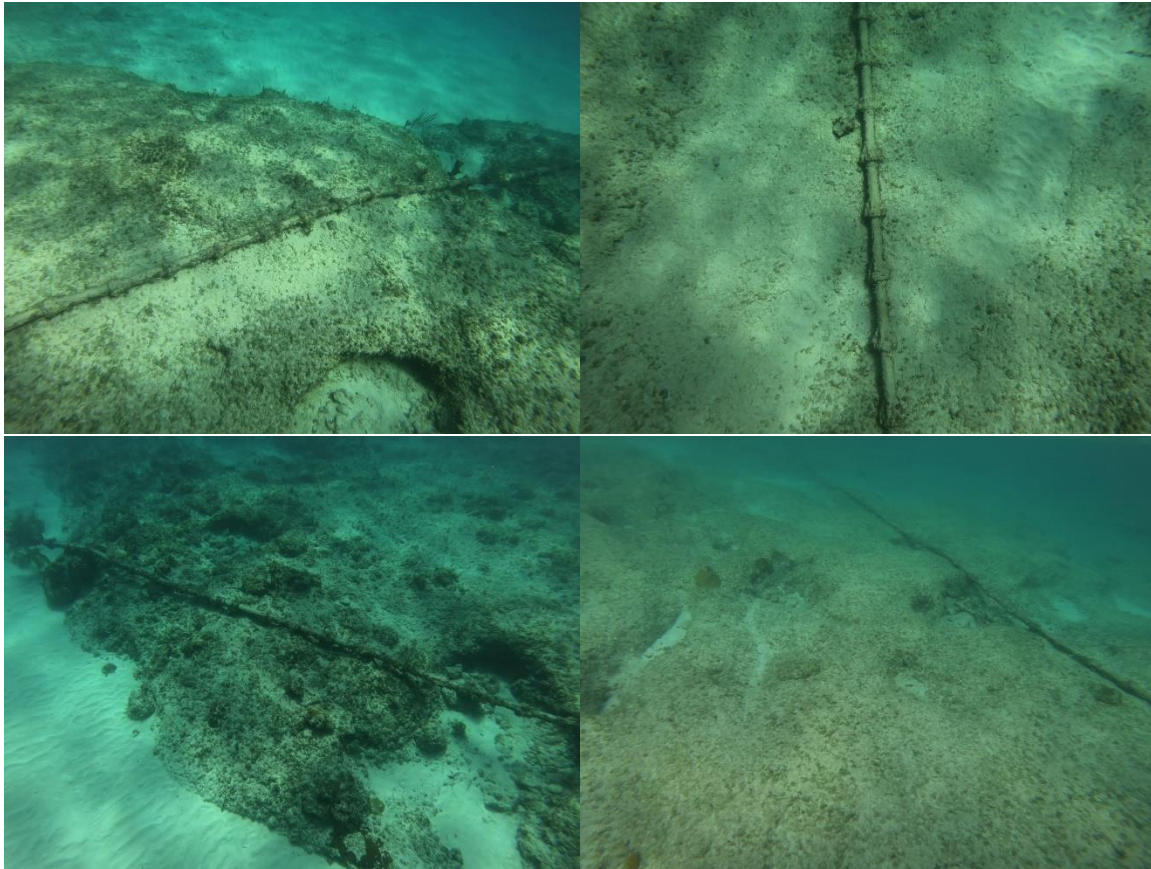
Figure 7.162. Images of subaqueous ICT cable off the southern shore of Leeward Harbour (2018).
