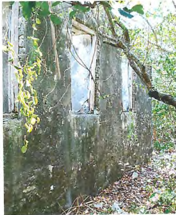
Figure 59, Barque Bay Structure 5, detail of north façade
