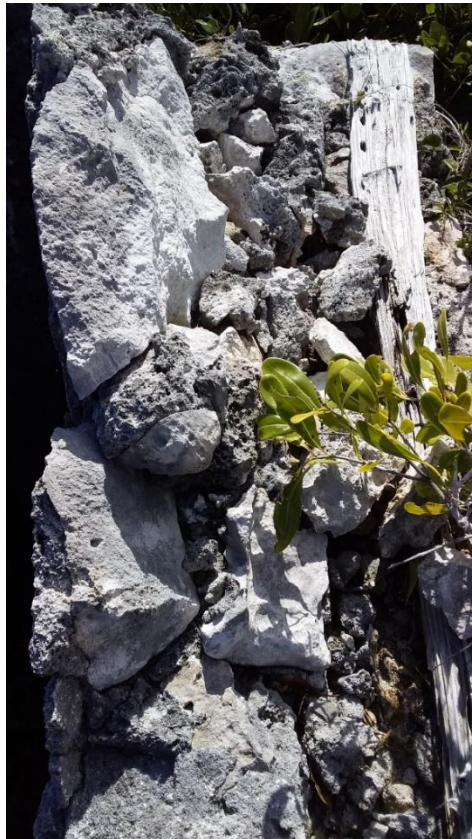
Figure 7.170 View of ruins at Barque Bay site
