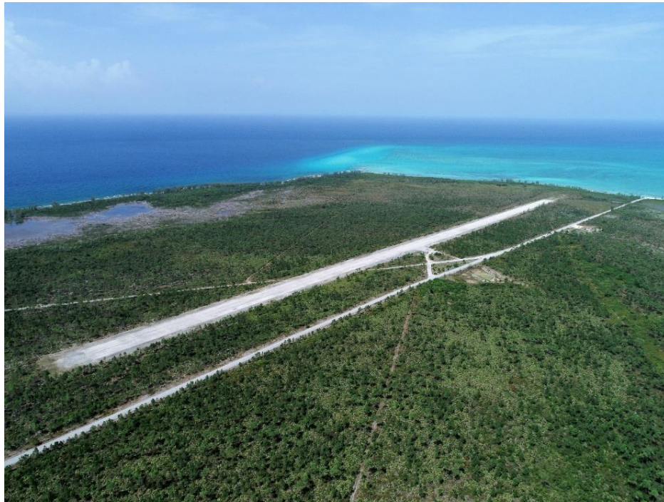
Figure 7.176. Sandy Point Airstrip with access road and Great Abaco Highway
