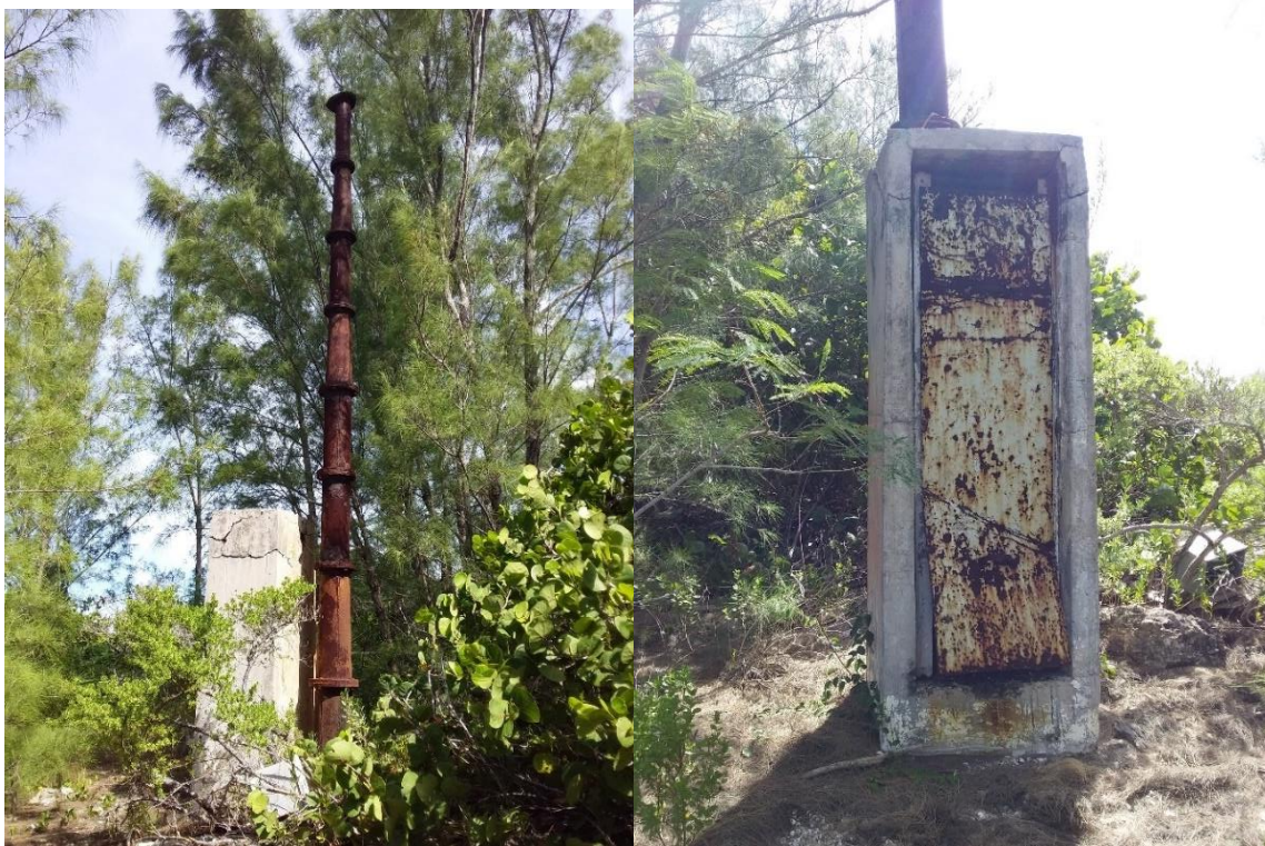
Figure 7.167. Remnants of Rocky Point 'lighthouse
