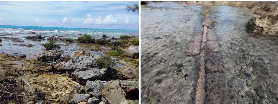
Figure 7.138 Black Mangrove among the rocky intertidal zone, Exposed cable (2018).
